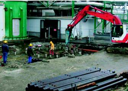
Grout Injection through the pile bore during driving
