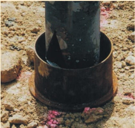
DYWIDAG Driven Ductile Iron Pile with grouted annulus page 6
