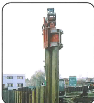
1500 meter sheet-piles (some double ones) in 8,5 hrs in Austria (only one operator needed)
