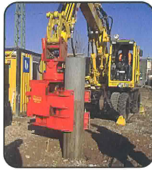
Movax SP 60W driving Ø 400-600 mm pipes on the German railway
