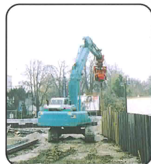
1500 meter sheet-piles (some double ones) in 8,5 hrs in Austria (only one operator needed)
