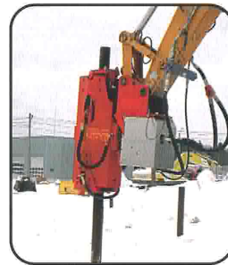
Movax TPH - foundation hammer - "PDA" can be seen on the monitor
