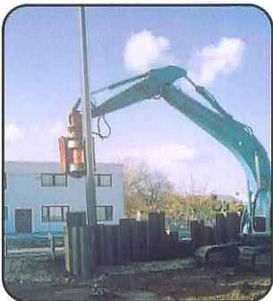
1500 meter sheet-piles (some double ones) in 8,5 hrs in Austria (only one operator needed)
